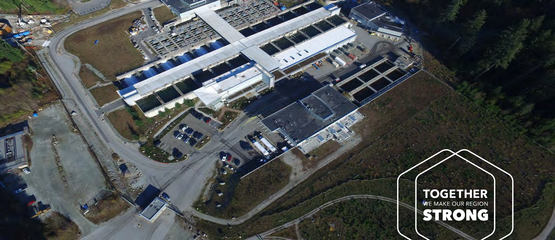
Seymour Capilano Filtration Plant
