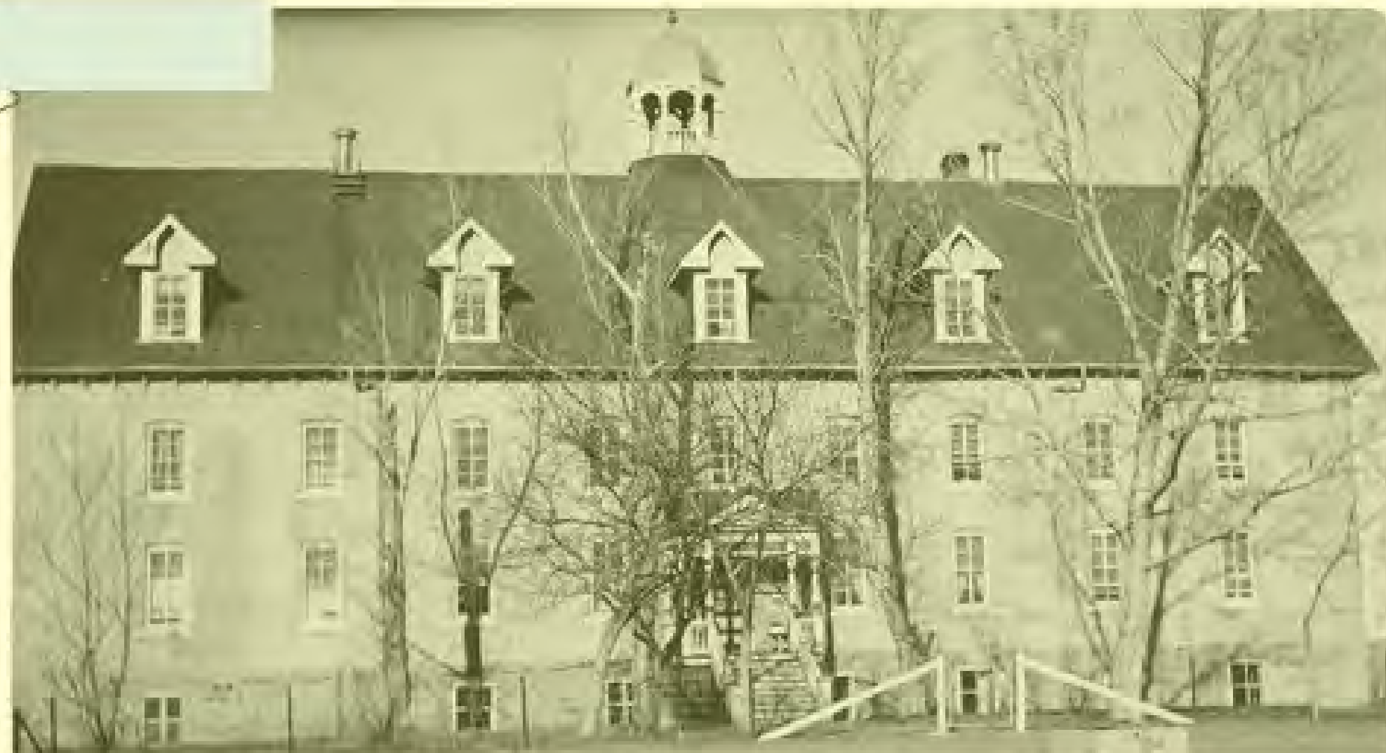
Marieval Cowessess Indian Residential School in Elcapo Creek Valley, Saskatchewan, n.d./ St. Boniface Historical Society Archives, 0001/SHSB 1461
